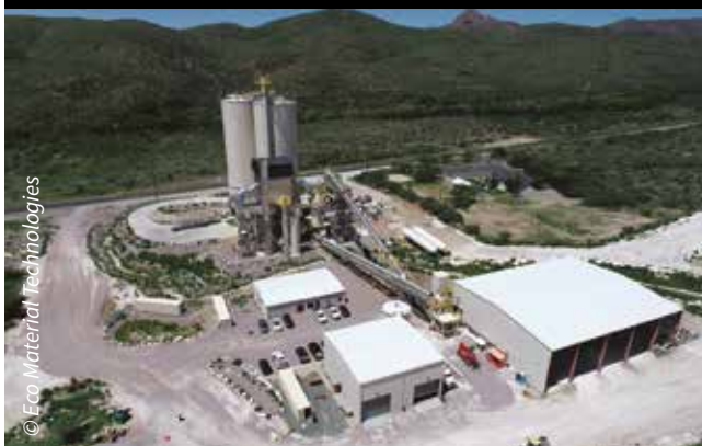
Eco Material Technologies Kirkland natural pozzolan plant in Arizona, USA
